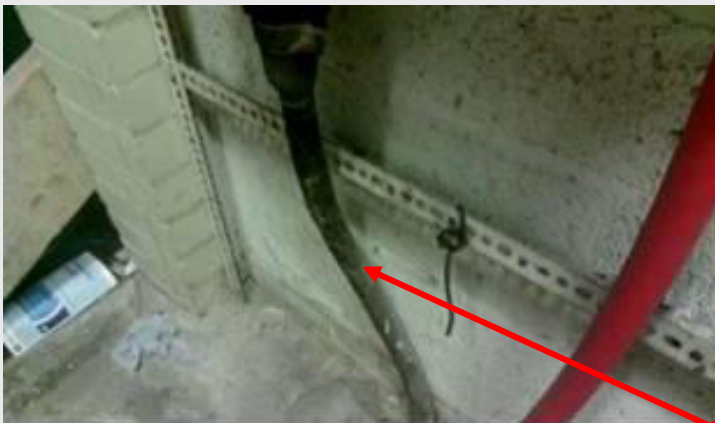
Wrap and bitumen coating
